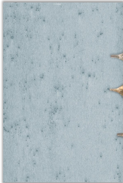
STAIRCASE COVE WALLCOVERING
